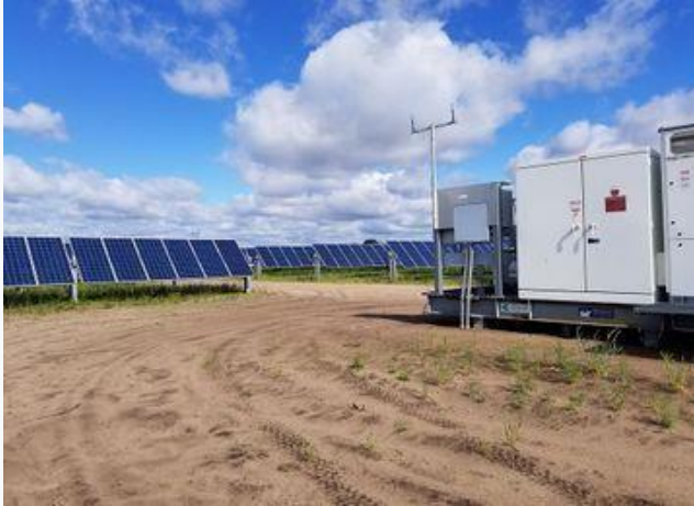
Figure 1. A photovoltaic system comprised of a solar panel array, inverter and other electrical hardware [1]
