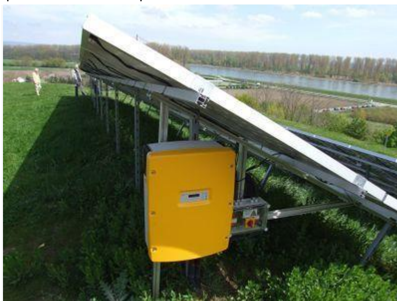
Figure 4. A solar inverter (yellow) mounted to the solar racking converts DC electricity from the solar array to useful AC electricity.
